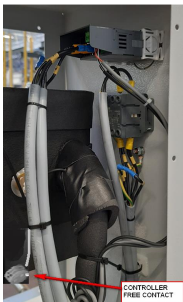
Location of the free contact connector for T60-125
