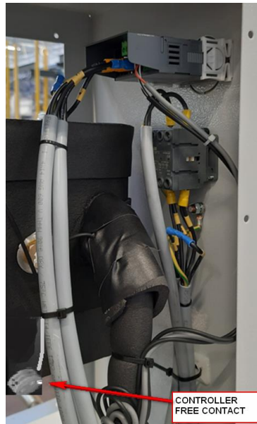
Location of the free contact connector
